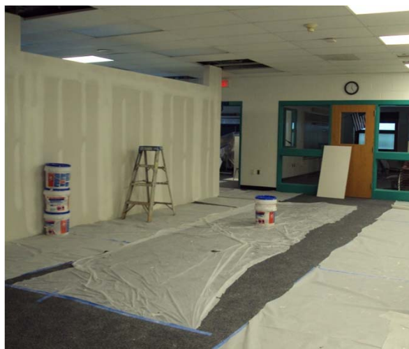
Construction of partition walls.
