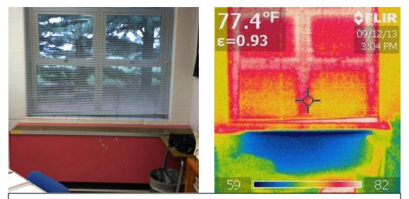
IR Photo of Room 31 Unit Ventilator and window. IR Photo shows heat infiltration at the window frame and window sill above the unit ventilator. Condensation was noted on the Unit Ventilator right side outer panel.
