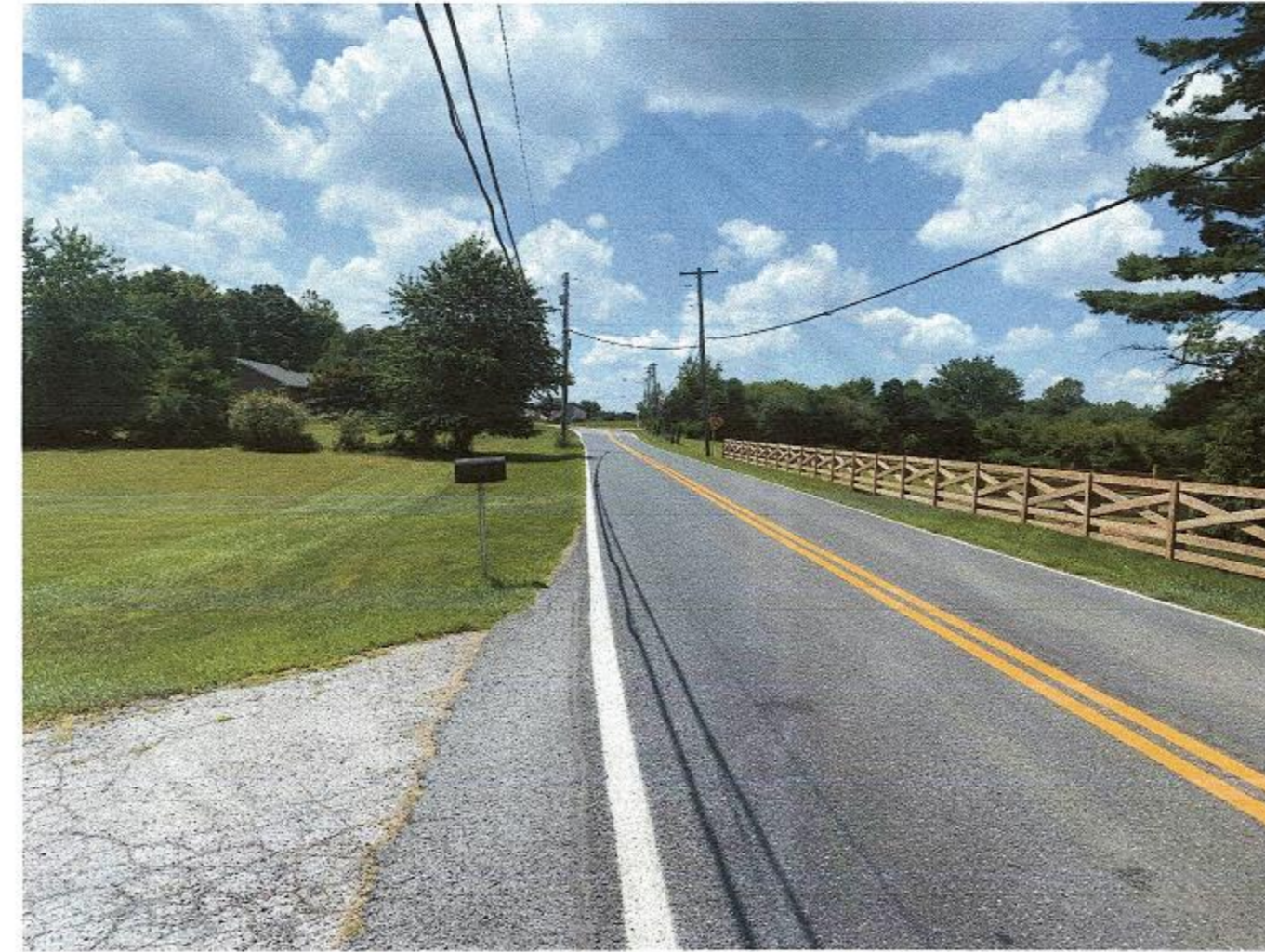
LONG CORNER ROAD TOWARDS PENN SHOP ROAD
