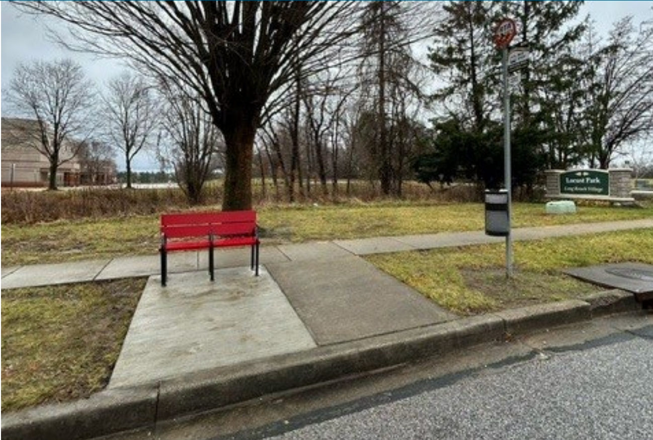
Tamar Dr. and Old Dobbin Ln. Larger ADA landing pad and bench
