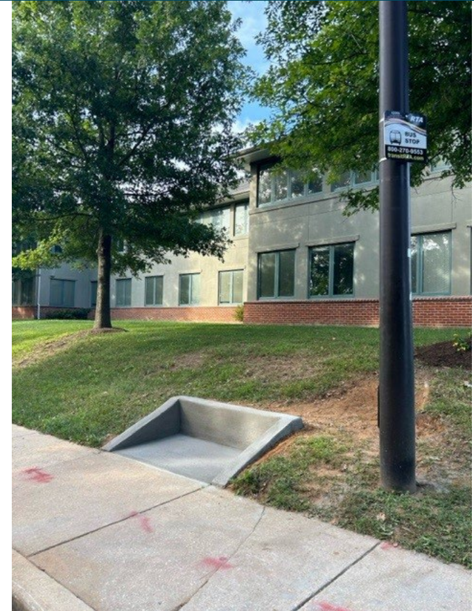
Freetown Rd. and Spring Step Knee wall makes the stop ADA
