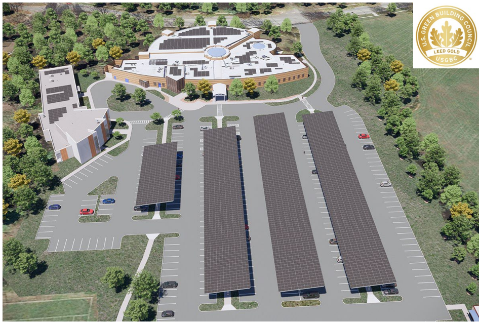
Solar canopies at East Columbia Campus
