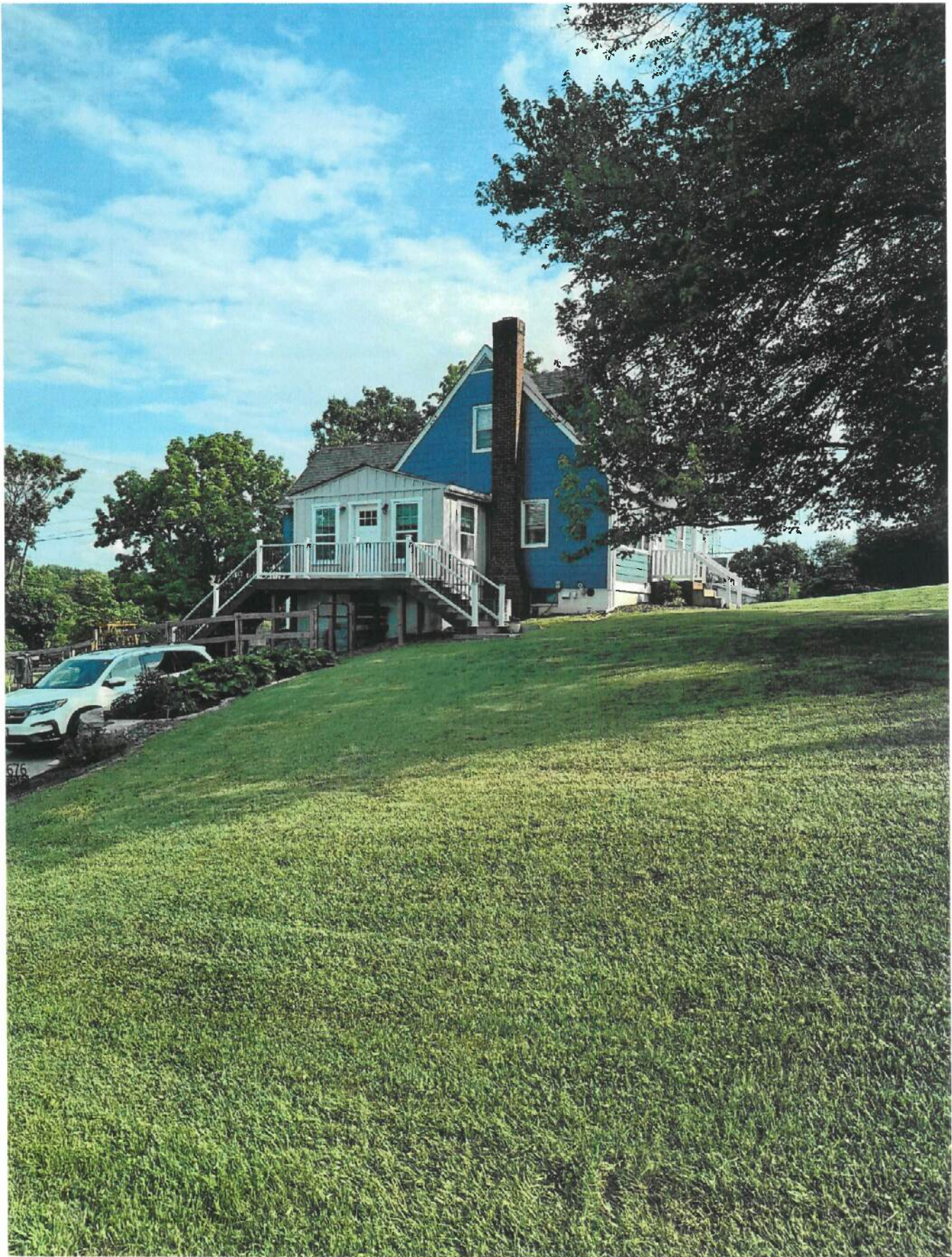
Street View of Finished Project Post Inspections these views are from the perspective of any neighbors that can see the stairs/landing.
