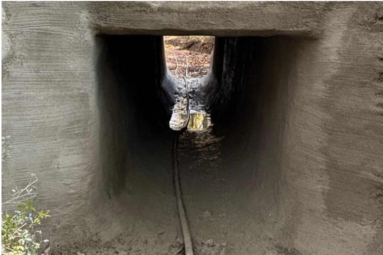
Ed Warfield Rd Culvert - After
