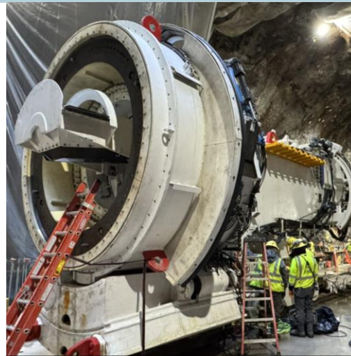
TBM Assembly – Mar 2026
