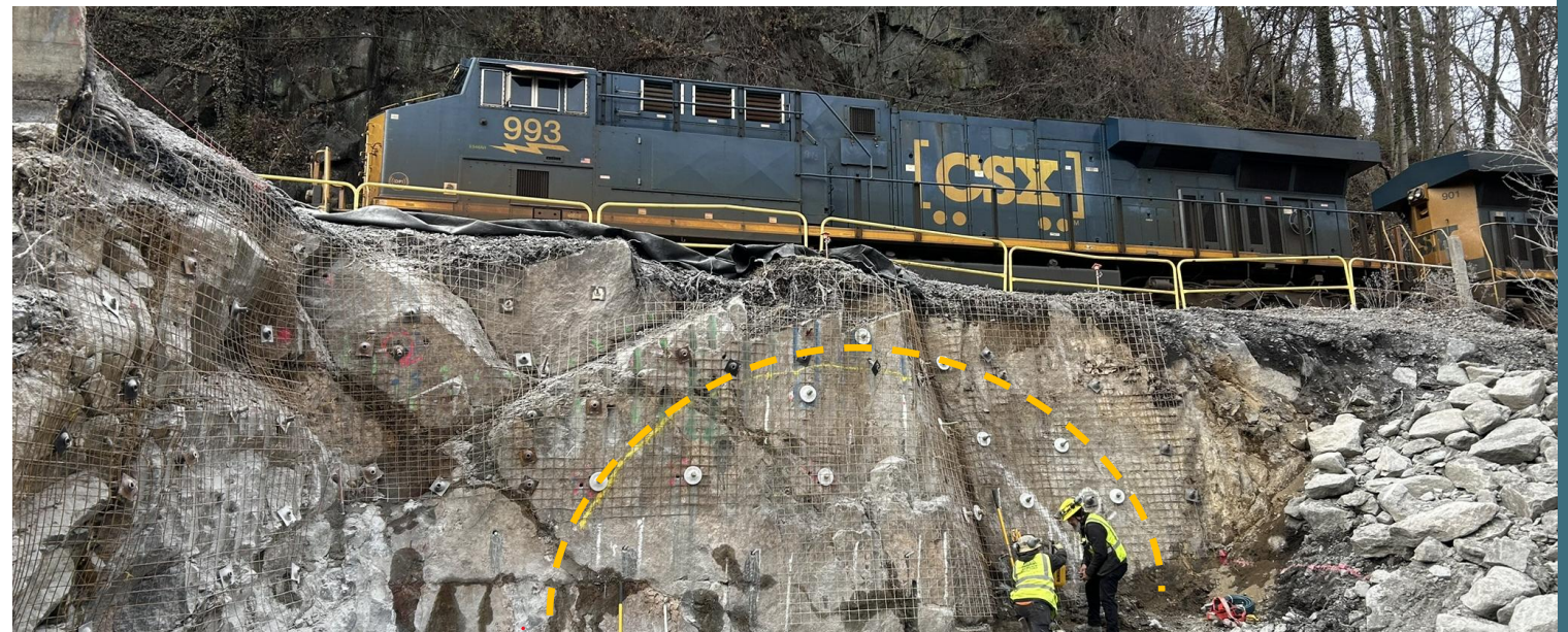
Patapsco Outfall – Feb 2026
