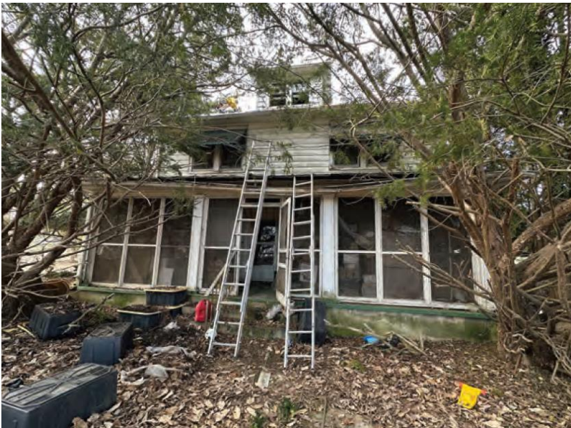
Figure 29 - Front of main historic house; to be demolished.
