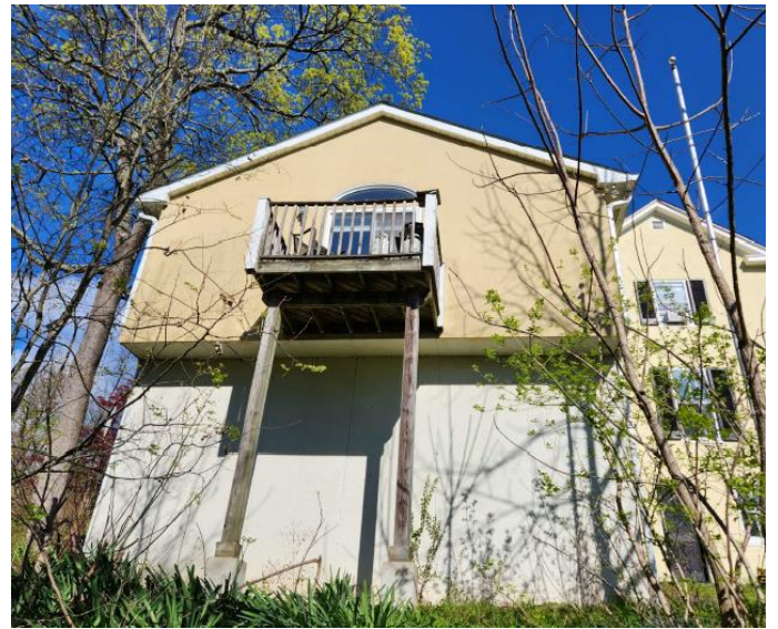
Figure 8 - Existing south (rear) elevation.
