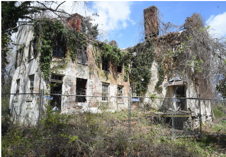
Figure 20 - Rear of John Holland house, photo date 2021.
