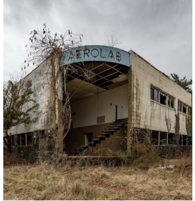
Figure 23 - Image of Aerolab exterior.
