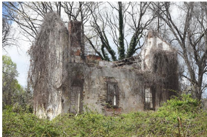
Figure 19 - Front of John Holland House, photo date 2021.
