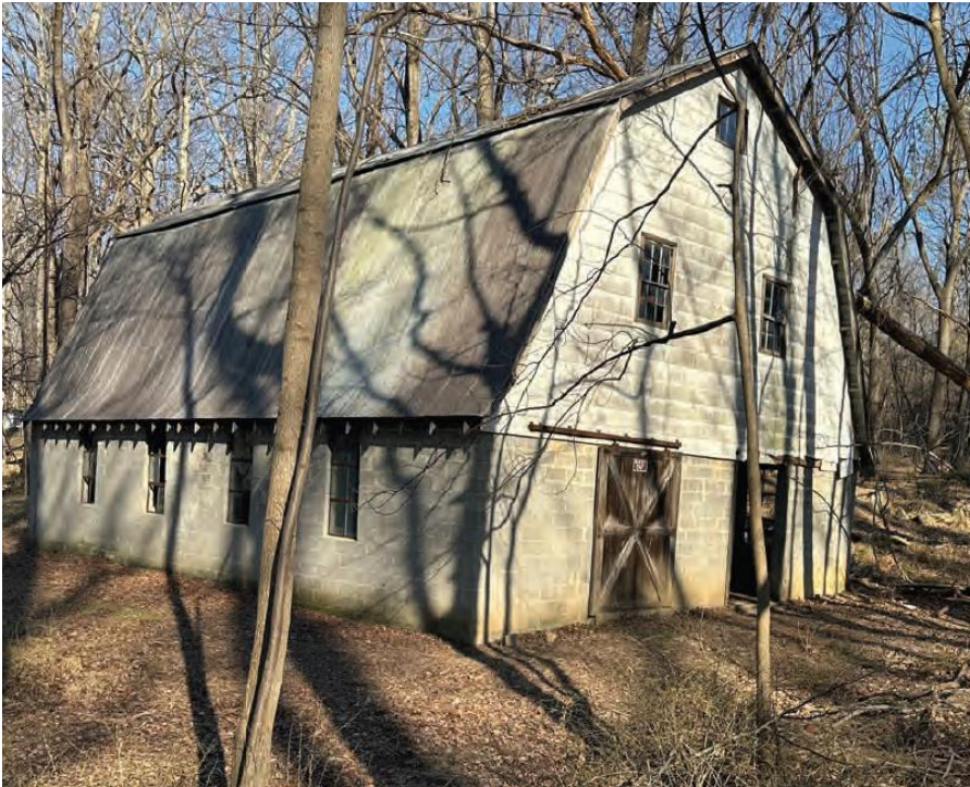
Figure 33 - Existing barn to be demolished.
