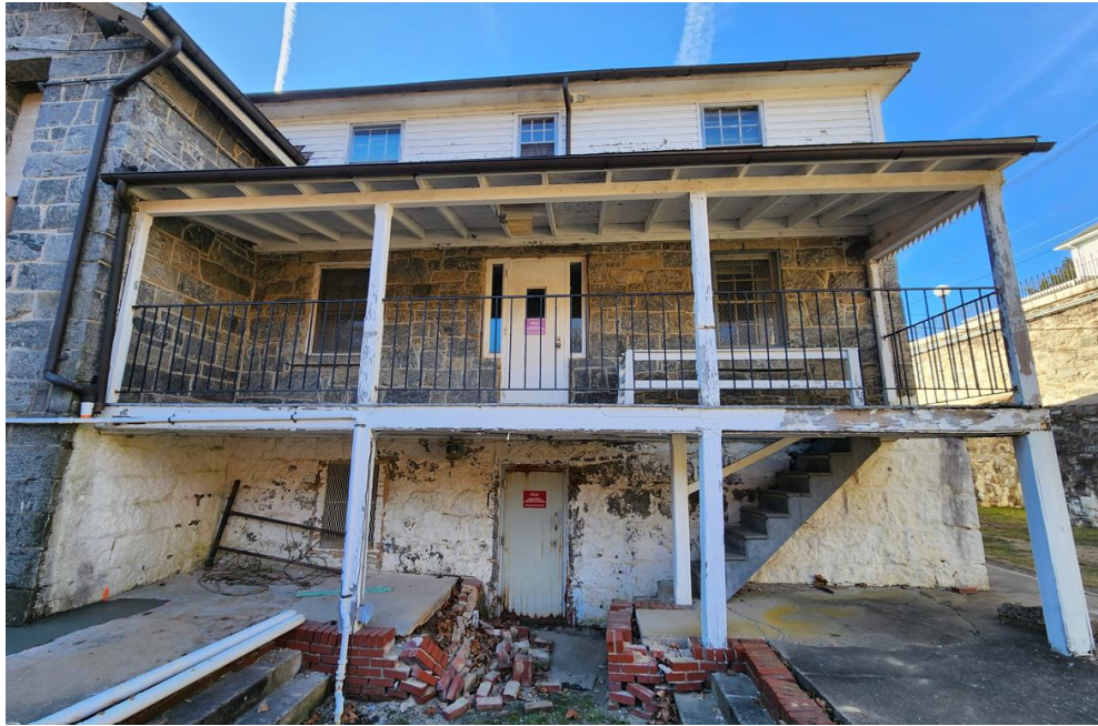
Figure 50 - Image of 1910/1851 section of building; existing conditions.
