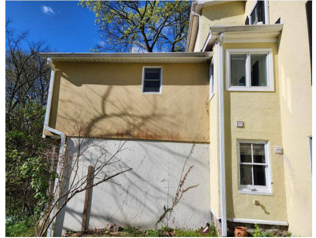
Figure 10 - Existing east (left) elevation.
