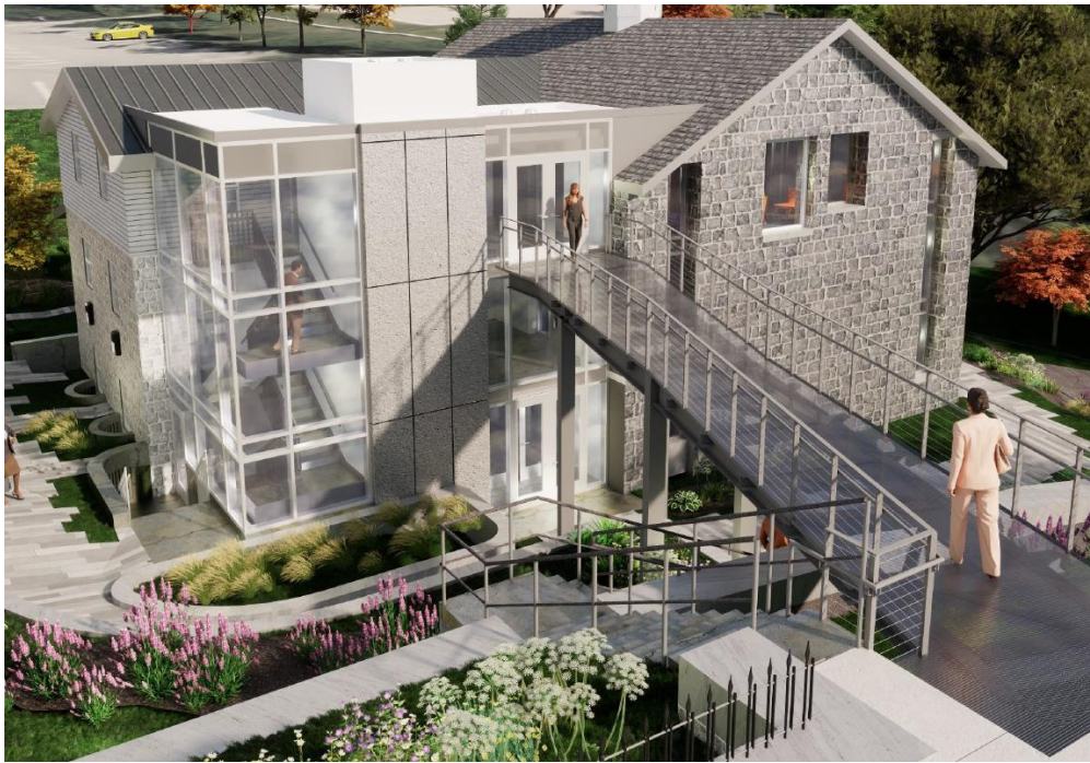
Figure 41 - Rendering showing proposed addition with aluminum and glass curtain wall system and stone panel wall system.
