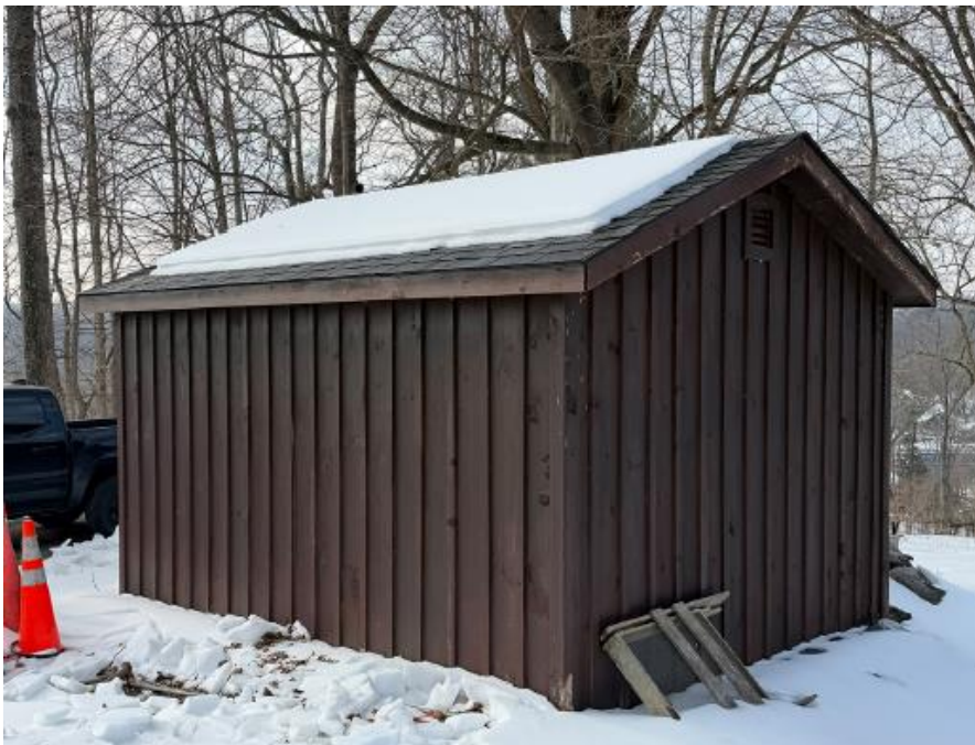
Figure 1 - View of existing shed.
