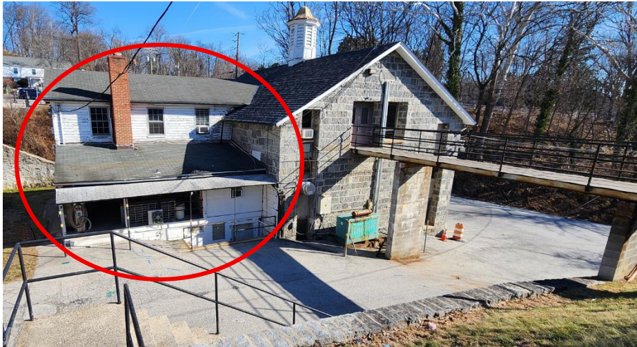
Figure 35 - Image of 1952 addition and pedestrian bridge proposed for demolition.
