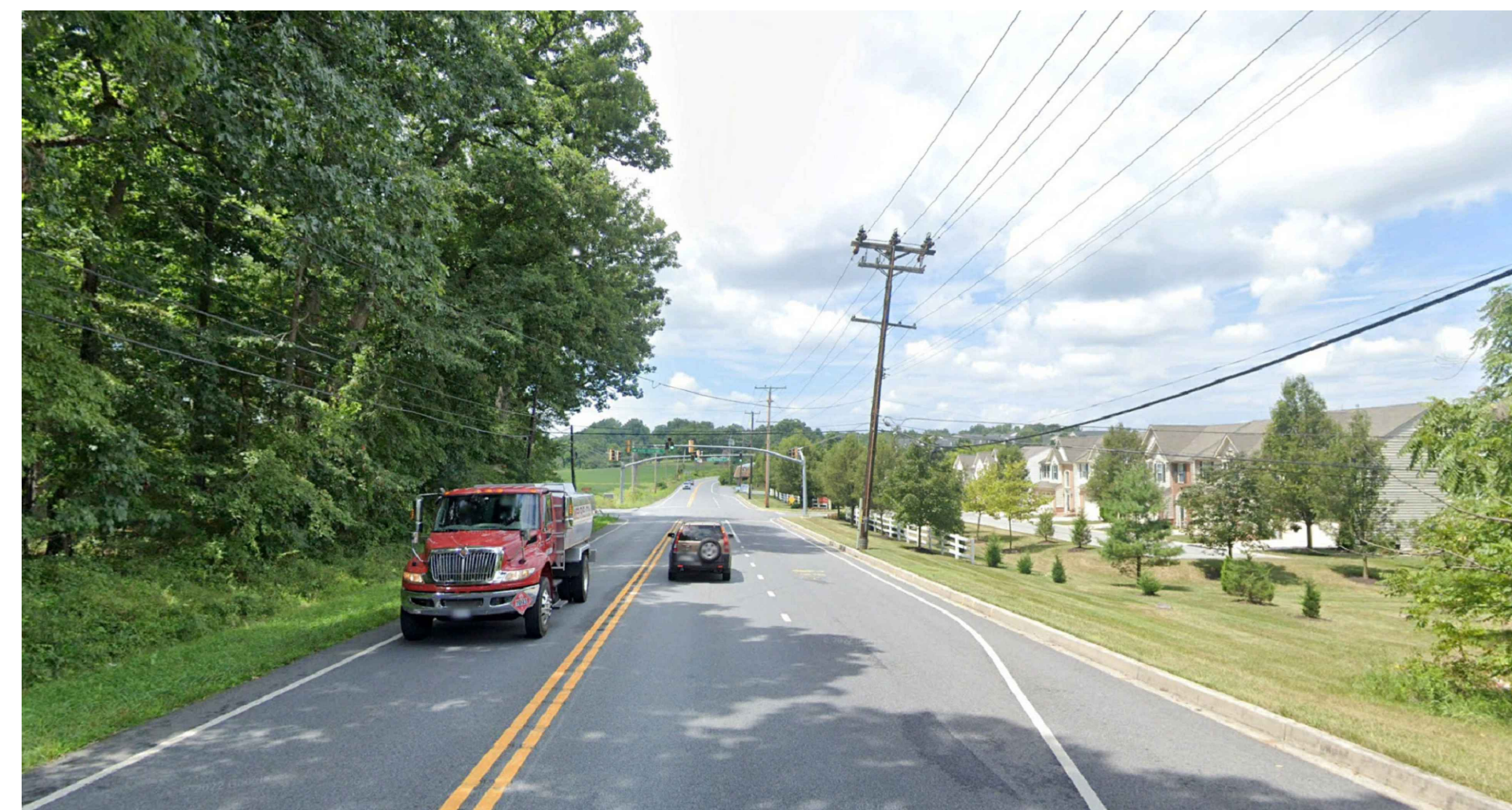
PROJECT ENTRANCE LOOKING WEST
